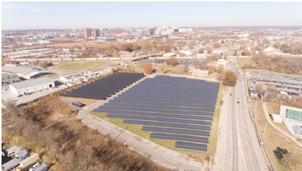
Figure 3: This picture denotes the 500 kW bifacial panel expansion on the Western side of this picture. Bifacial panels create a better aesthetic and are more durable panels than monofacial panels.
