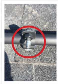
Photo 7: Where not protected from physical damage, equipment grounding conductor must be #6 or larger: NEC 690.46, 250.120(C). Conductors laying on asphalt shingles will become damaged and will not last a PV system's expected 30-year lifespan.
