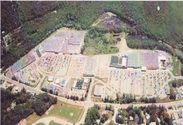
The Cortlandt Town Center along Route 6 is one of the few regional retail centers in northern Westchester County.
