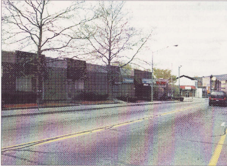
Redevelopment of the Crossroads Plaza in Downtown Peekskill was identified as an opportunity to improve the area's vitality.
