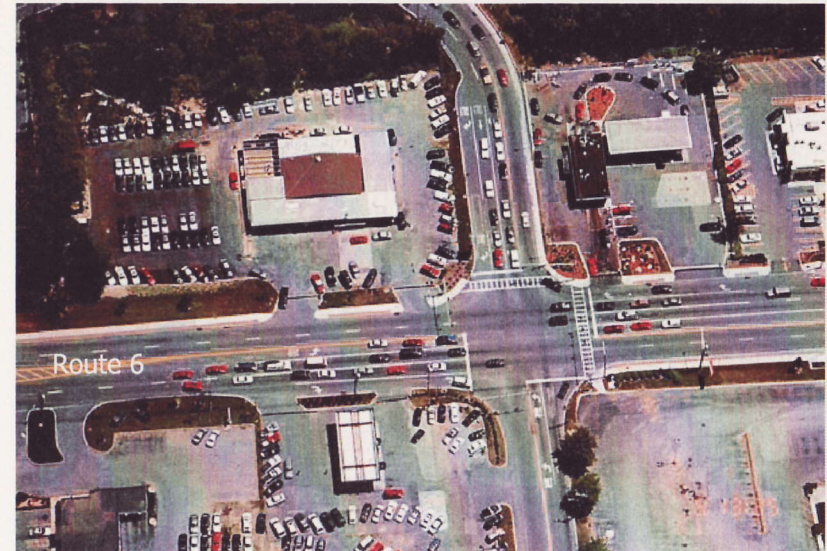
The intersection of Route 6 and Westbrook Drive is scheduled for a series of improvements.
