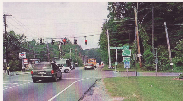
Bear Mountain Parkway route sign needs to be relocated.
