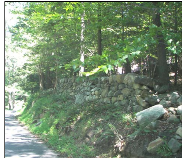
Stonewall along Hunterbrook Road, Hunterbrook.
