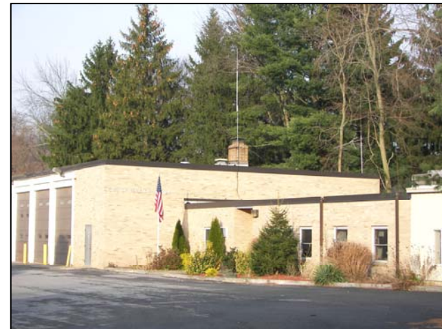
Town of Yorktown Water Department.
