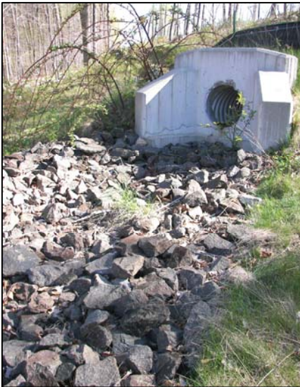
A drainage outfall.
