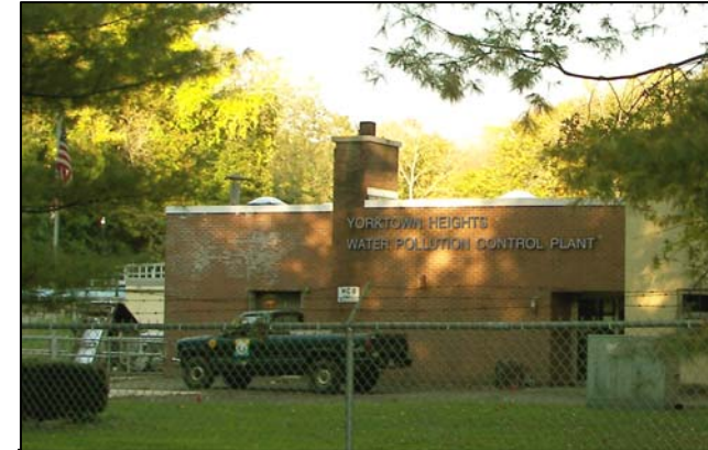
Yorktown Heights Water Pollution Control Plant, Greenwood Street, Yorktown Heights.
