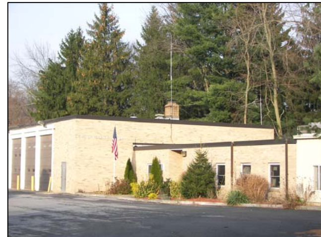
Town of Yorktown Water Department.
