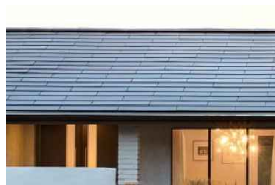
B Tesla Roof Street View
