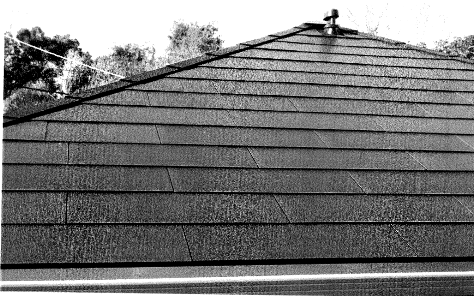
TYPICAL ROOF TEXTURE
