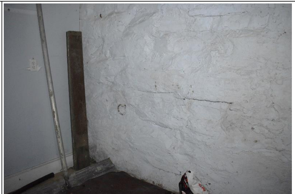
#10. The northern foundation wall of Building E is the 19 th century stone barn wall, consisting of field stone that has been painted.
