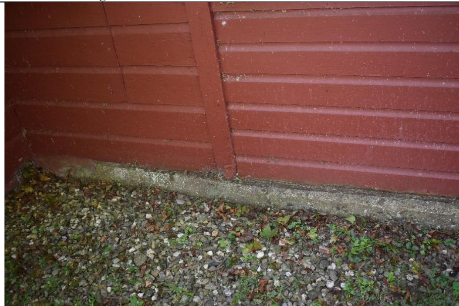
#35. Building H is located on a poured concrete slab.
