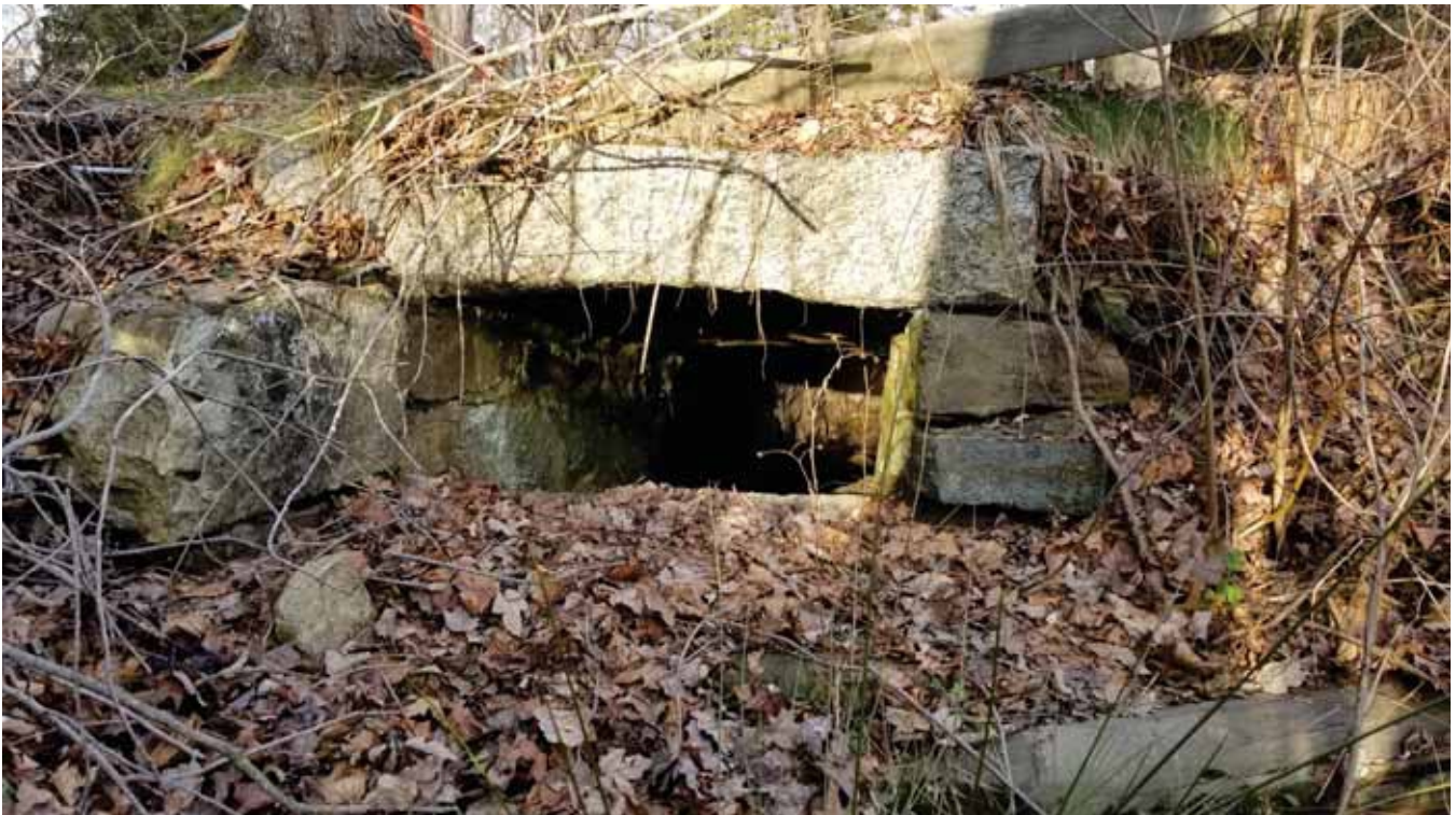
Photo 4 - Existing Pond Outlet
