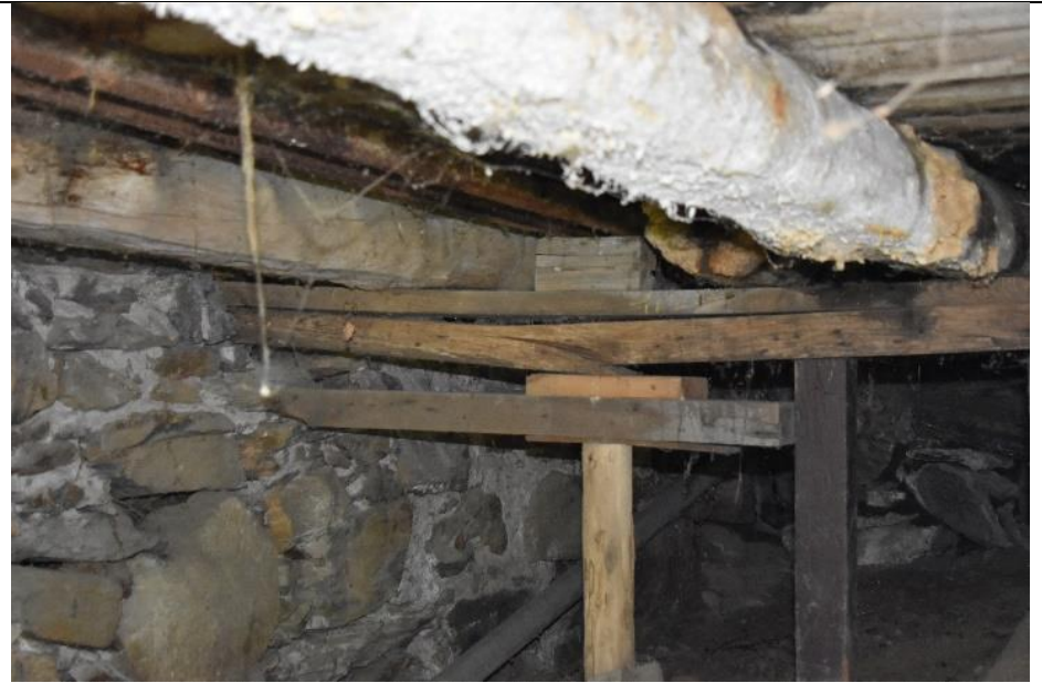
# 26. The foundation and barn supports are a mix of timber, early 20 th and 21 st century lumber. The beams underneath the main floor of Building G are rotted.
