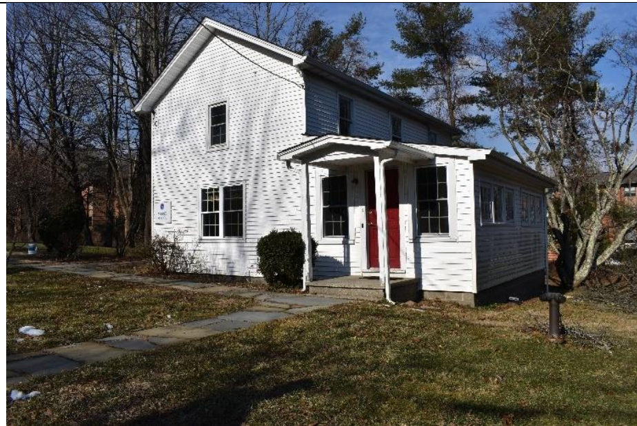
#7. The exterior of Building C includes modern vinyl siding.
