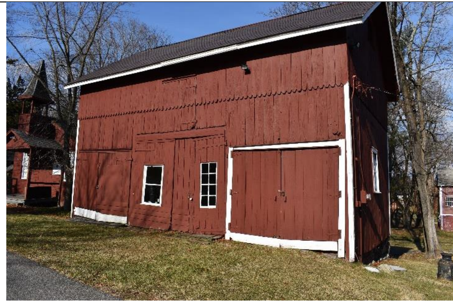
#21 View northwest of Building G, the entrances and openings have been modified over time.
