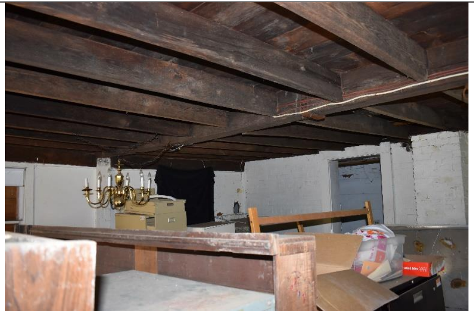
#42. The interior of Building J is a mix of brick and cut lumber, that appears to be early 20 th century.
