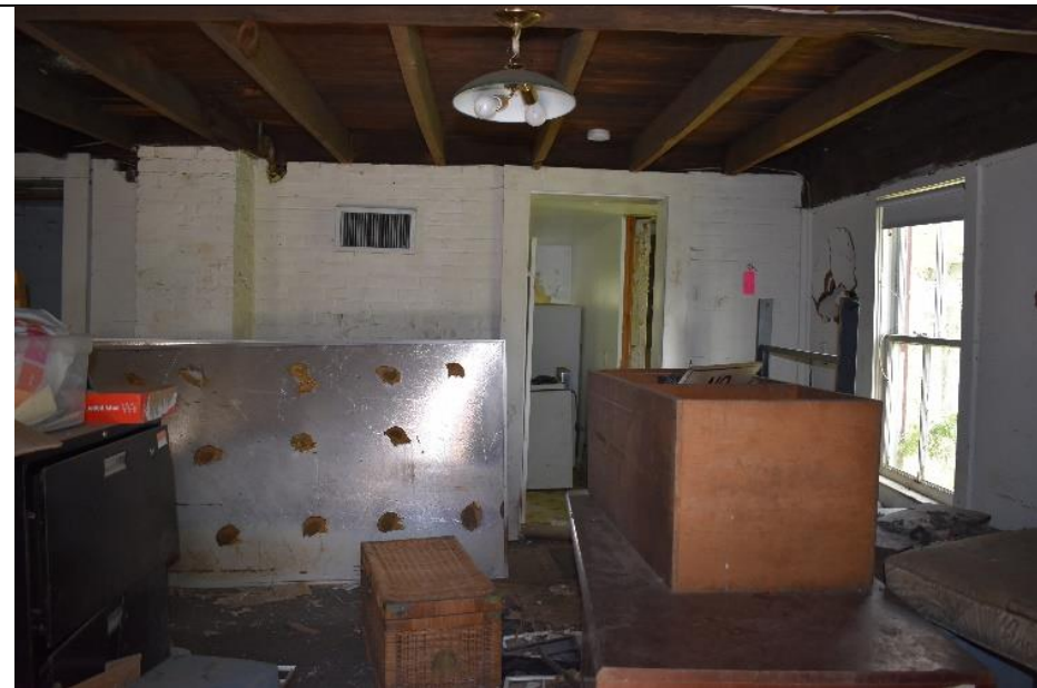
#43. A brick wall divides the interior of Building J.
