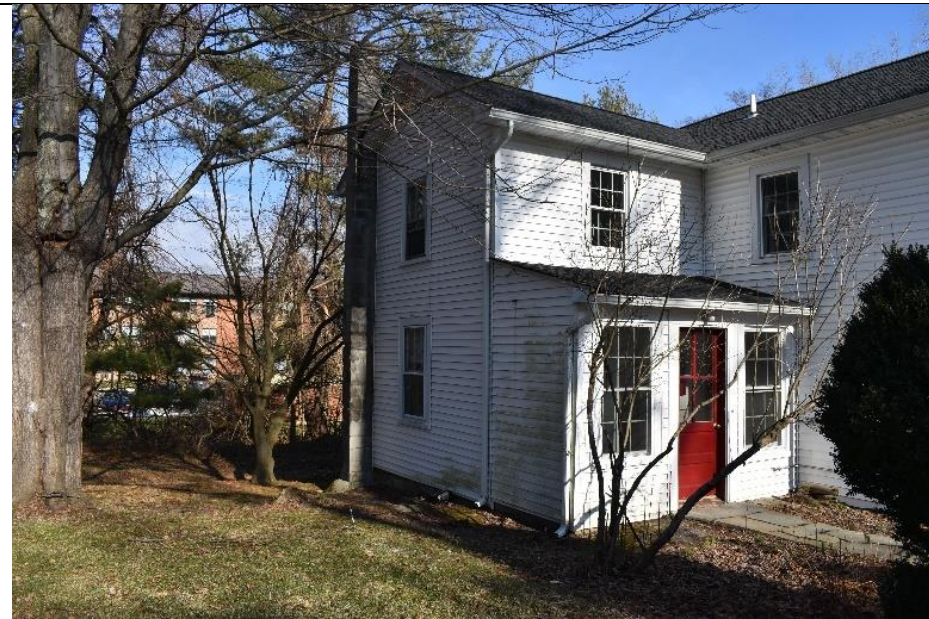
#8. The western entrance of Building C features an enclosed doorway addition.
