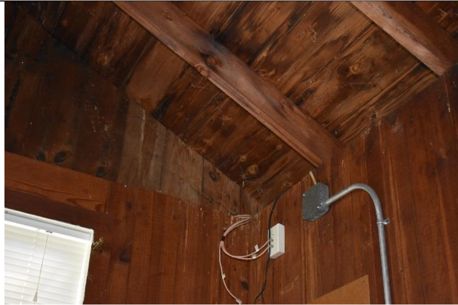
#33. The interior features platform framing and 20 th century construction materials Building H.
