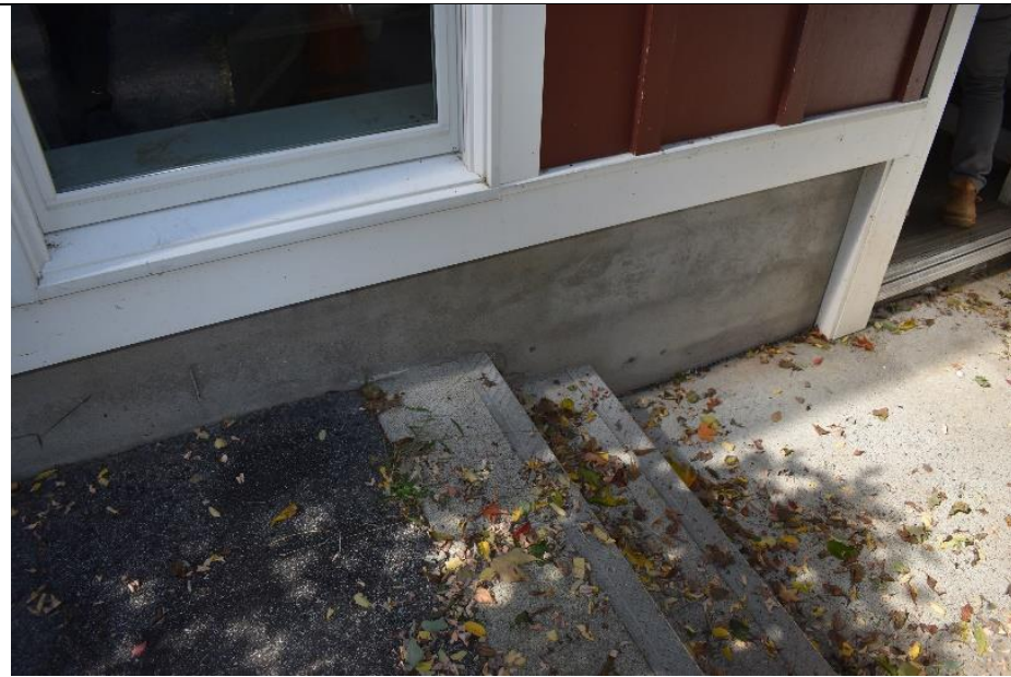
#9. Building E features a modern concrete foundation on the southern and eastern walls.
