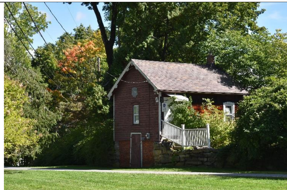
#1. View to the northeast to Building B.
