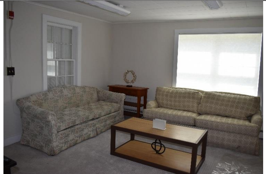
#6. The interior of Building C was recently renovated.
