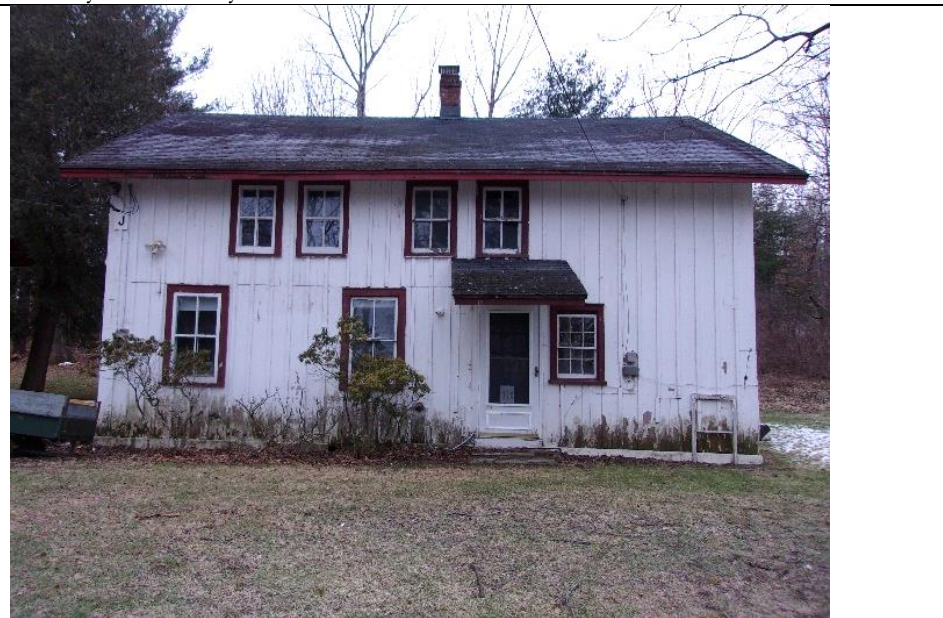
#44. The fenestration on the exterior of Building J is uneven, and the windows are mixed in size, and pattern.
