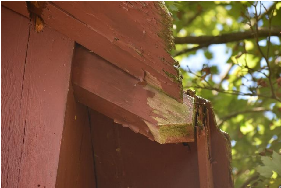
#27. The mix of lumber styles (clapboard, plywood, boards) is visible on the exterior of Building G's roofline.
