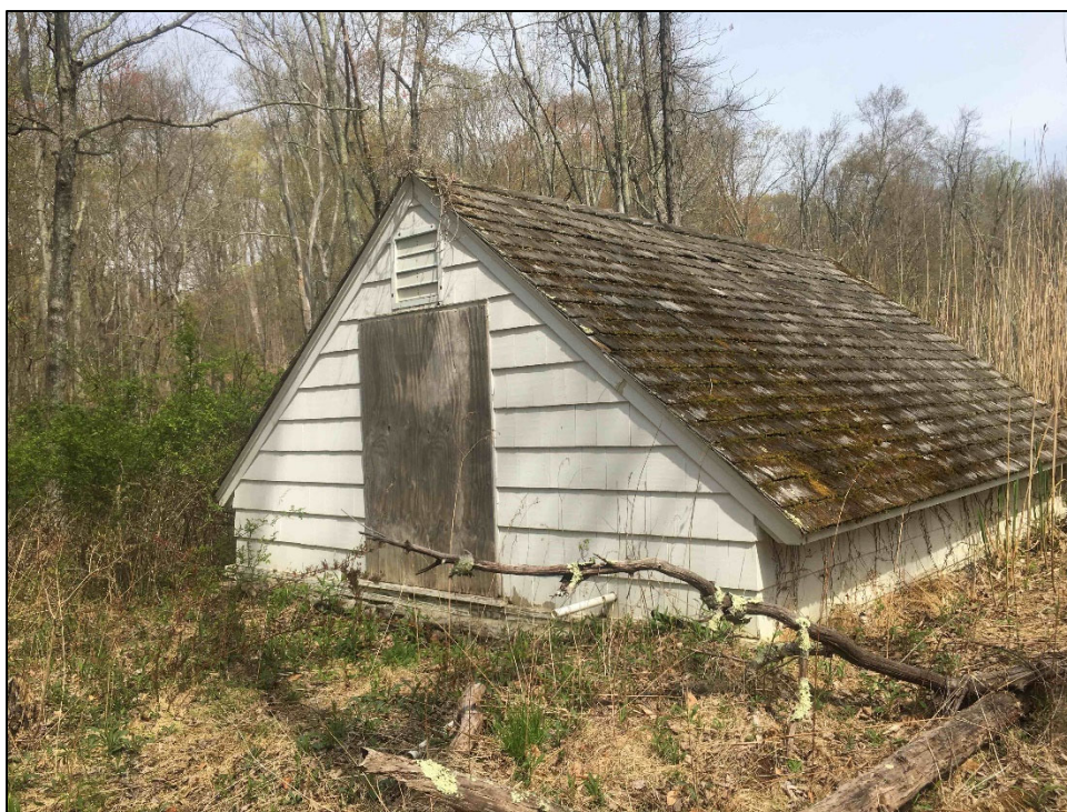
16. Overview of well house observed, facing northwest.
