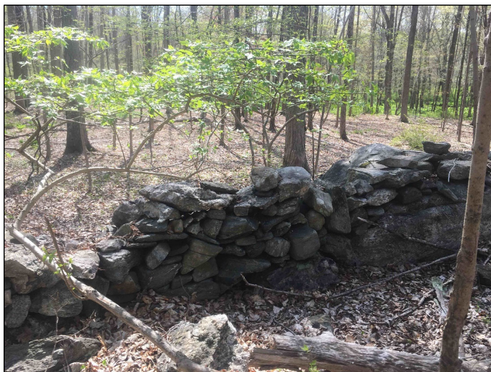
14. Overview of rock wall, facing southeast.
