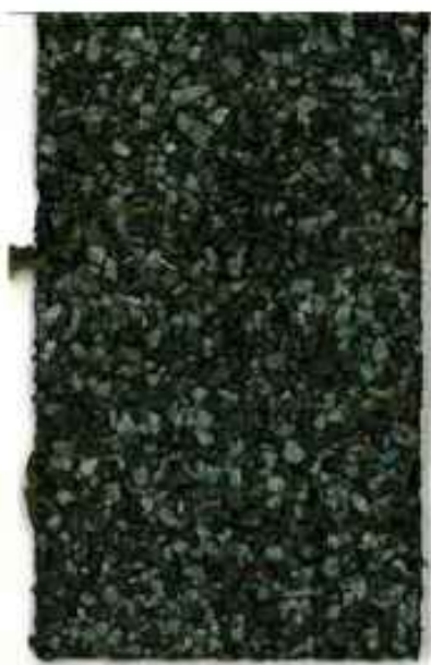
R1 - ASPHALT ROOF SHINGLES
