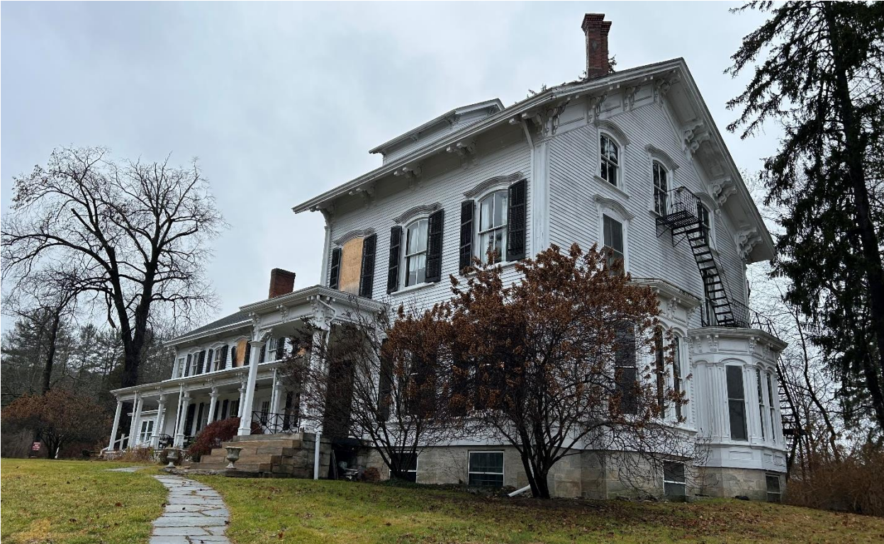
Figure 2. Photograph of Existing South & East Façades.
