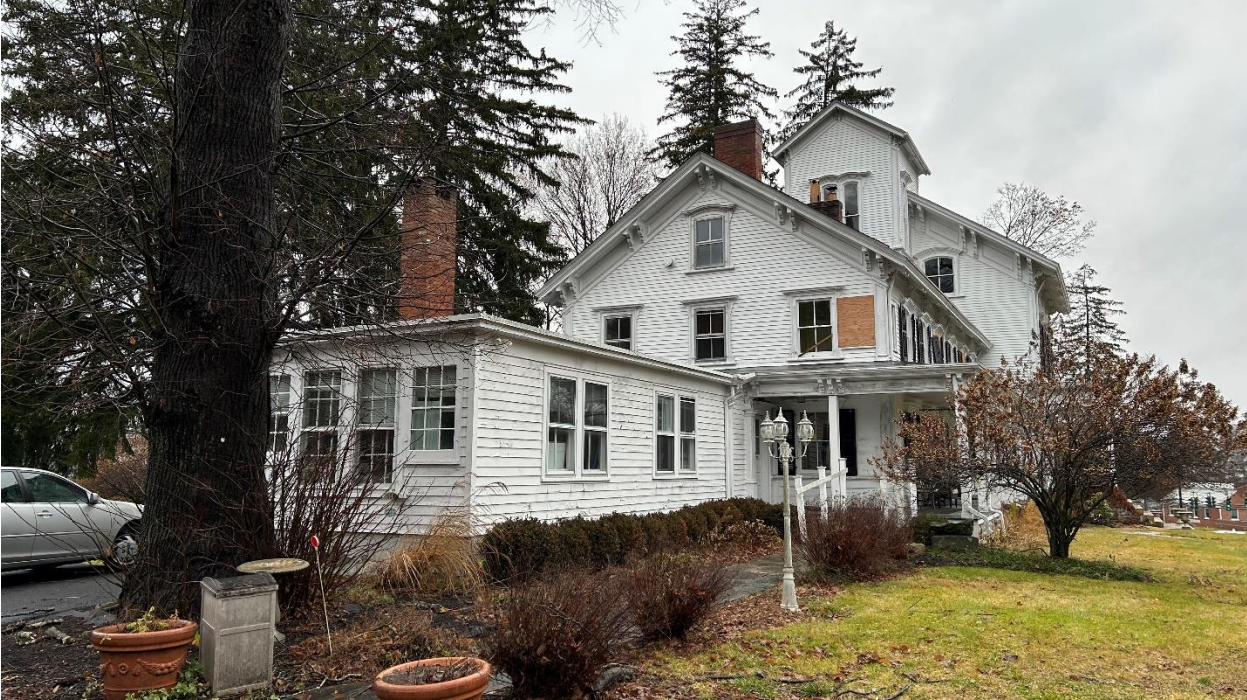
Figure 3. Photograph of Existing West & South Façades (Area of Proposed Porch Addition)
