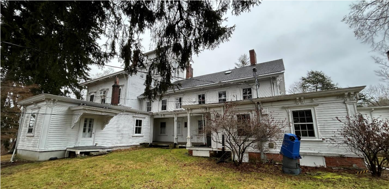
Figure 5. Photograph of Existing North Façade (Area of Proposed Kitchen Addition)
