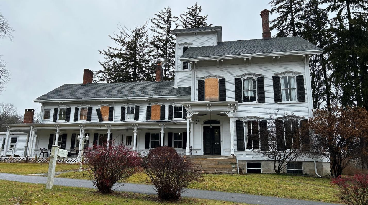
Figure 1. Photograph of Existing South Façade.
