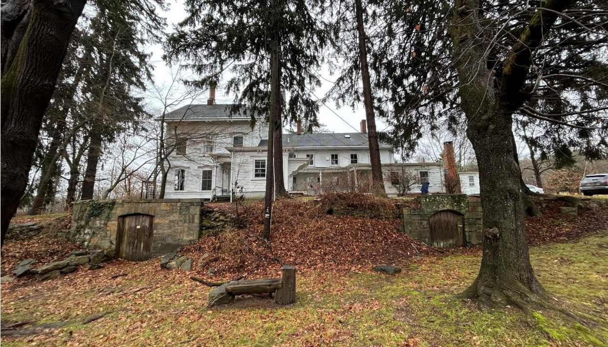
Figure 6. Photograph of Existing North Façade
