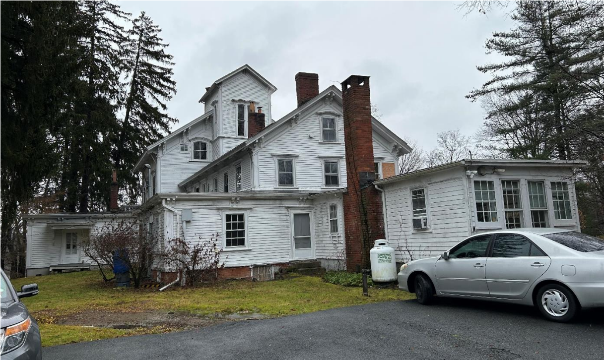
Figure 4. Photograph of Existing West & North Façades (Area of Proposed Kitchen Addition)
