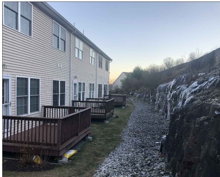
REAR OF UNITS NORTH SIDE
