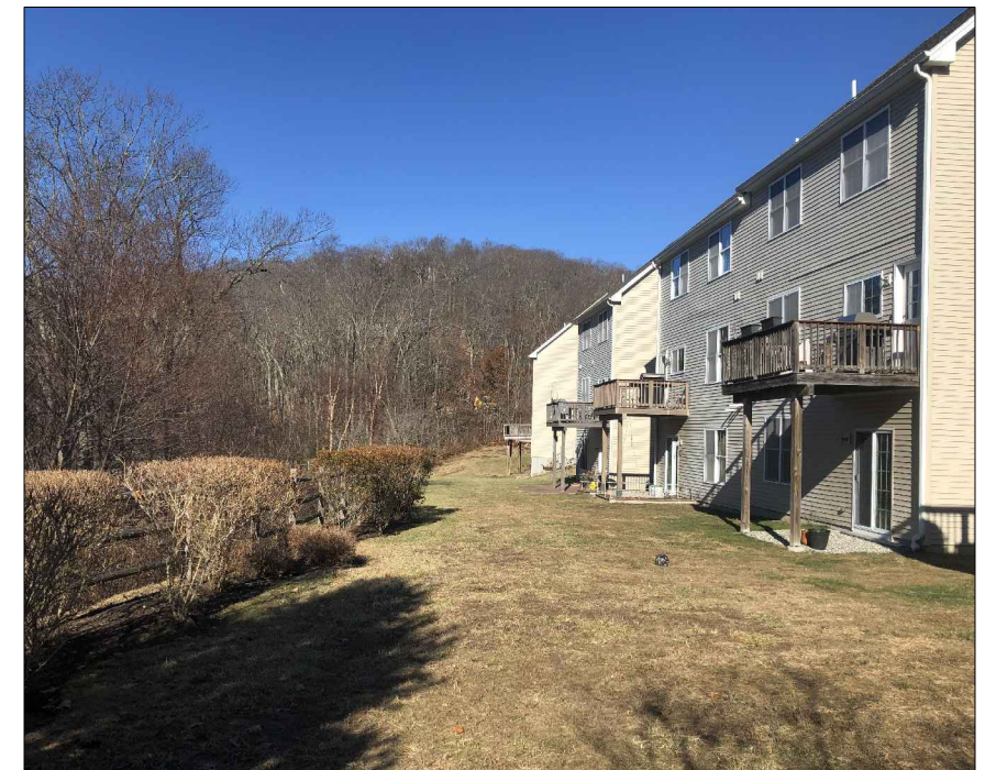
REAR OF UNIT SOUTH SIDE
