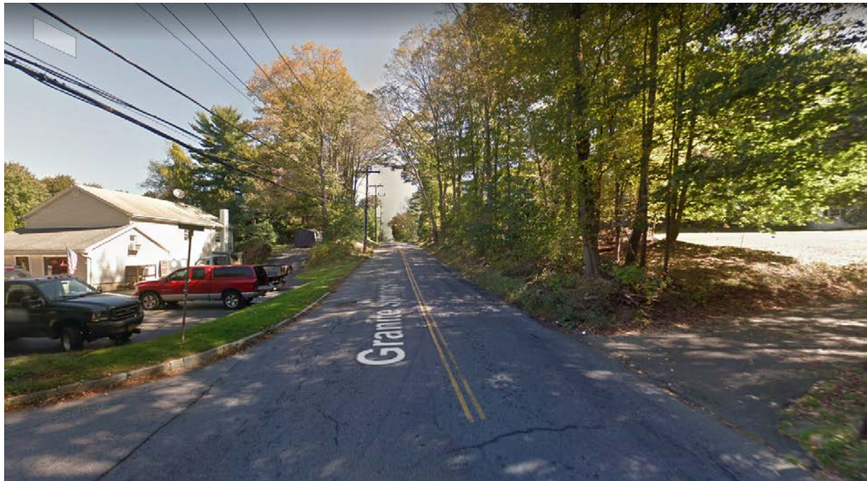
Photo 1. Granite Springs Rd and Gomer St intersection, facing east along Granite Springs Rd.
