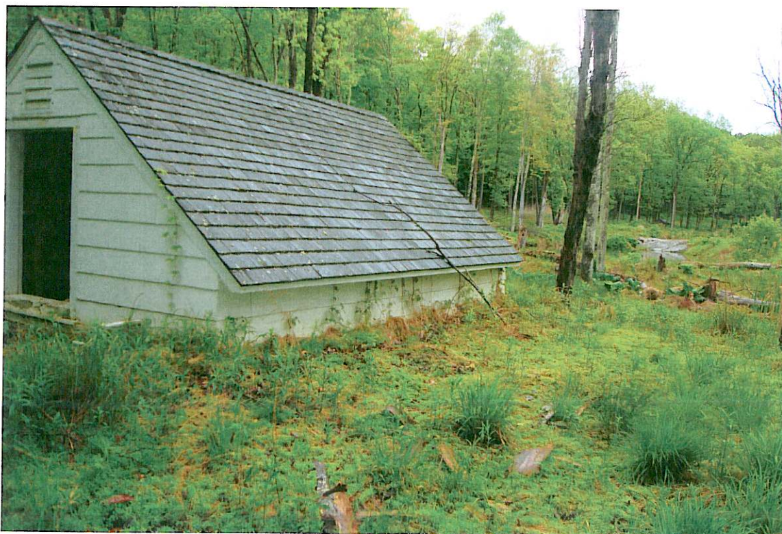
Photo No. 6 - North view/close up of on-site pump house just south of on-site ponds.
