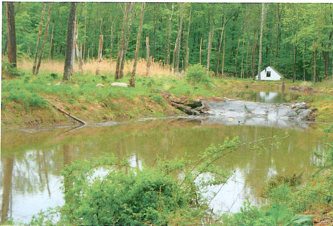
Photo No. 5 - South view of on-site ponds with pump house depicted in background.
