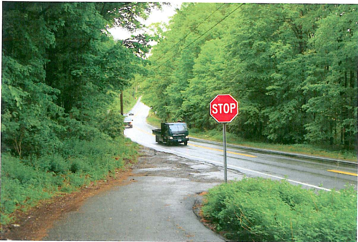
Photo No. 8 - View of Dell Avenue south intersection with NYS Route 100.
