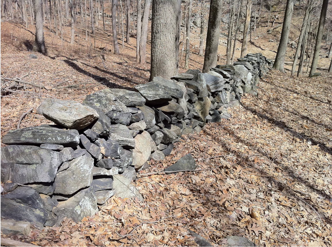
Stone Walls - Photo 2
