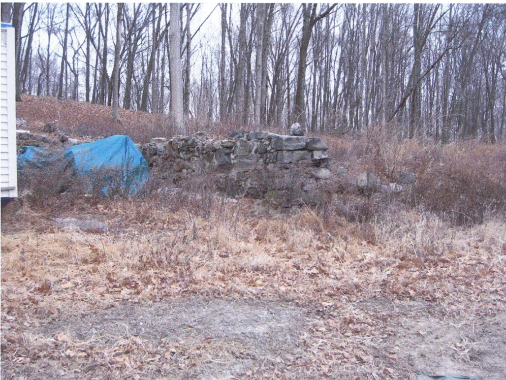
Photograph 21. Remnant of former 20th century outbuilding foundation.
