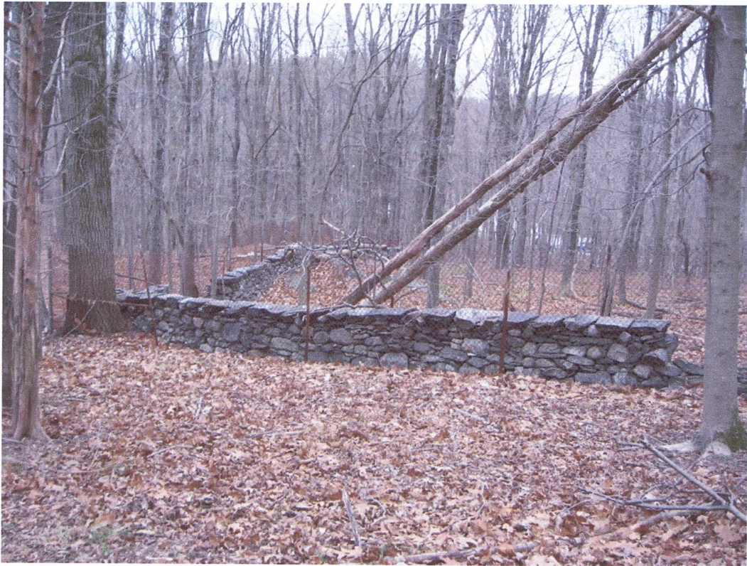
Photograph 3. Stone wall along Area 1.
