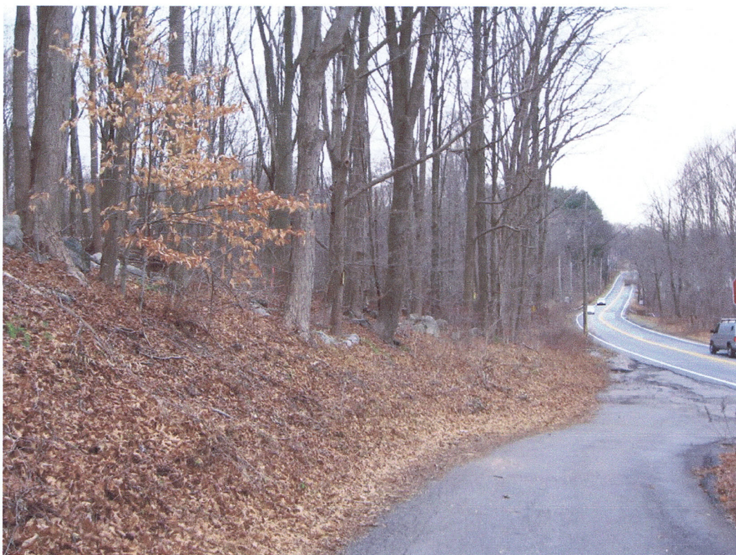
Photograph 6. Slope adjacent to Dell Avenue, west of Areas 2 and 3.
