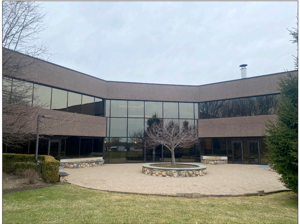
View towards north office building from within courtyard 7
