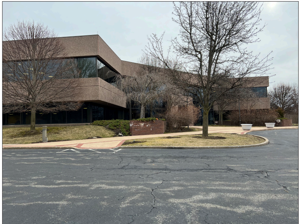
South office building 2
