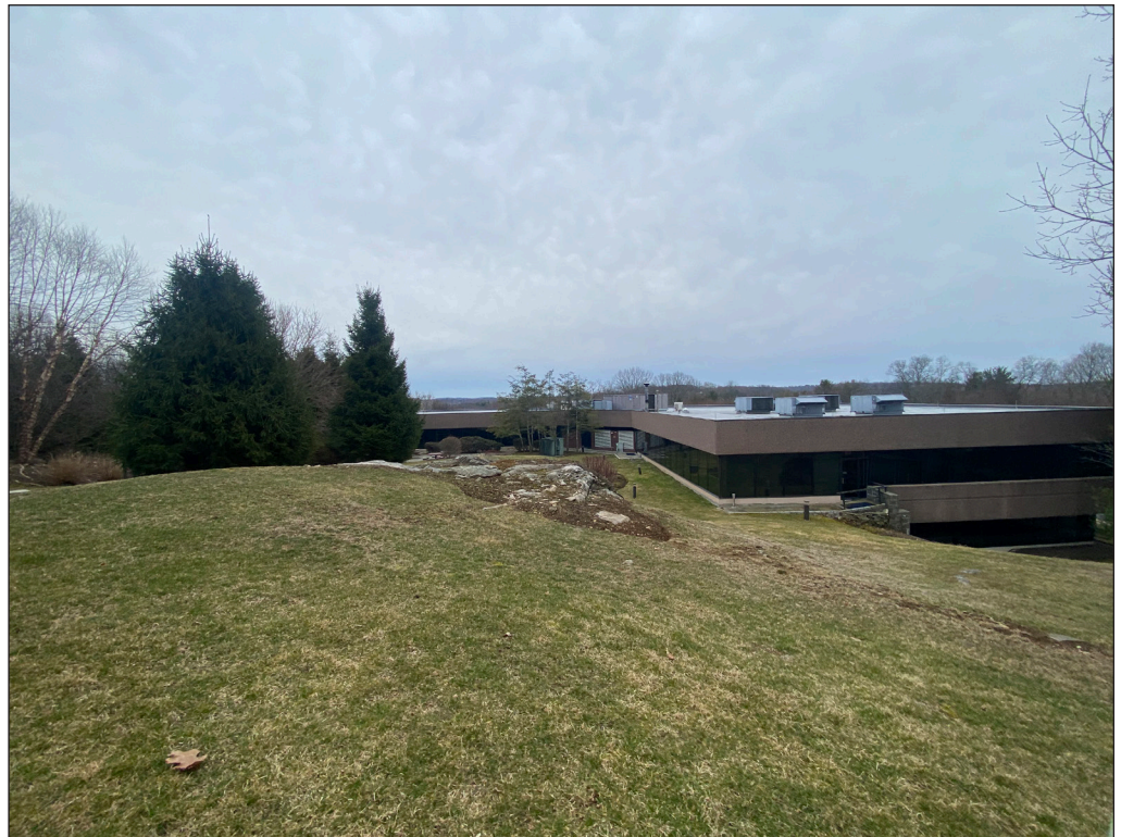
View from courtyard between office buildings looking toward south office building 6
