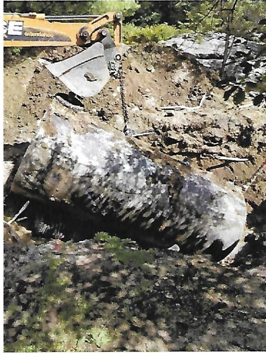
Photograph 1- Tank being removed from excavation.
