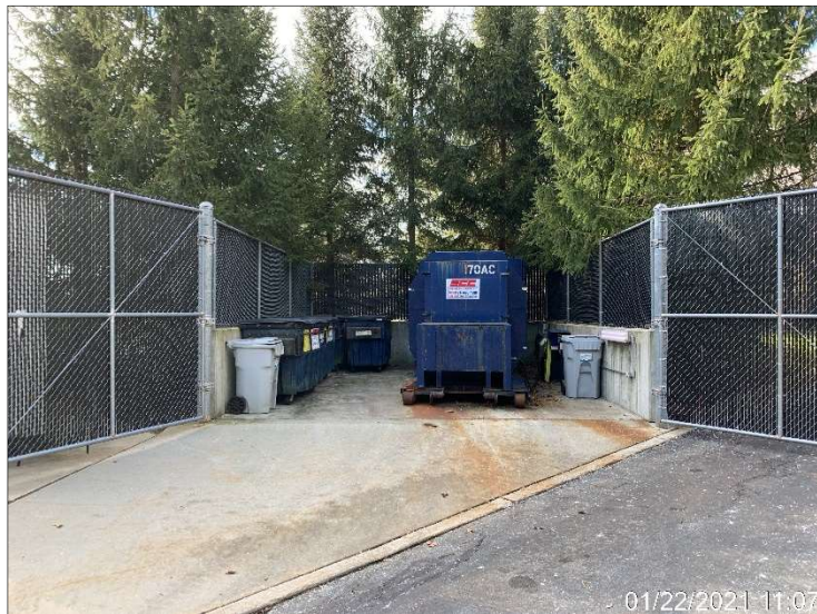
Photograph 31. Hydraulic compacting dumpster and several standard dumpsters for general refuse and recycling, located east of the office complex.
