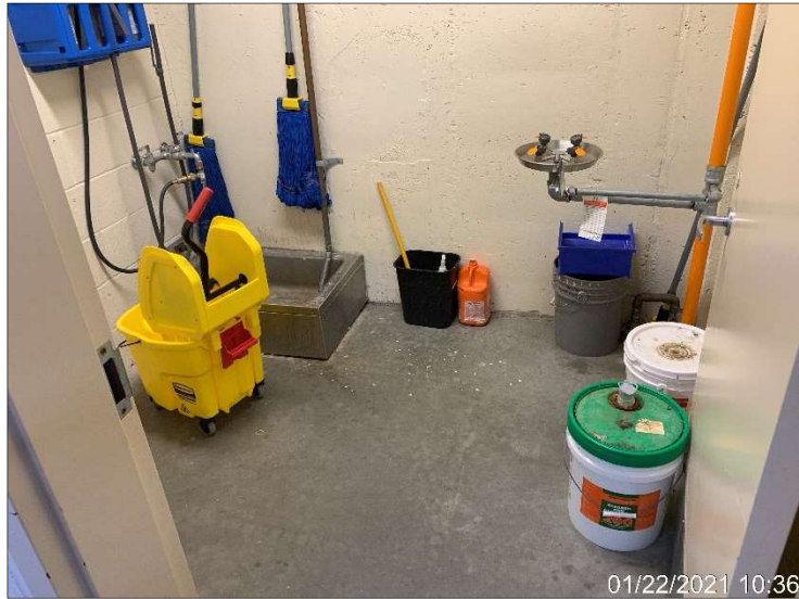
01/22/2021 10:36 Photograph 17. General cleaning supplies in the custodial storage room in the cellar of Building 2.
