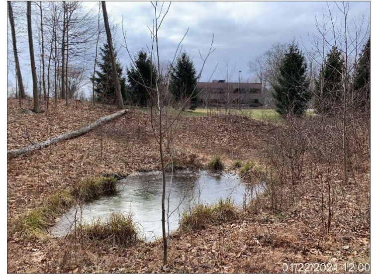
Photograph 34. Stormwater detention basin located north of the office complex.
