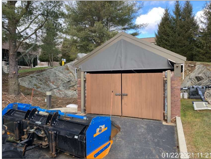
Photograph 25. Maintenance shed located east of the office complex. Note: bedrock outcrop.
