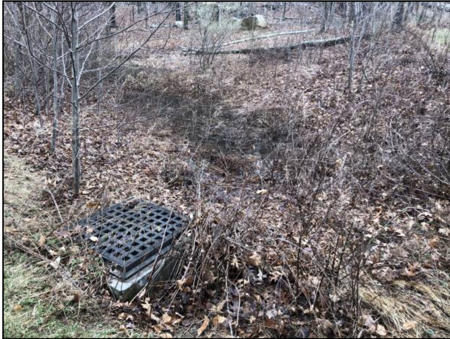
31 : Stormwater retention pond
