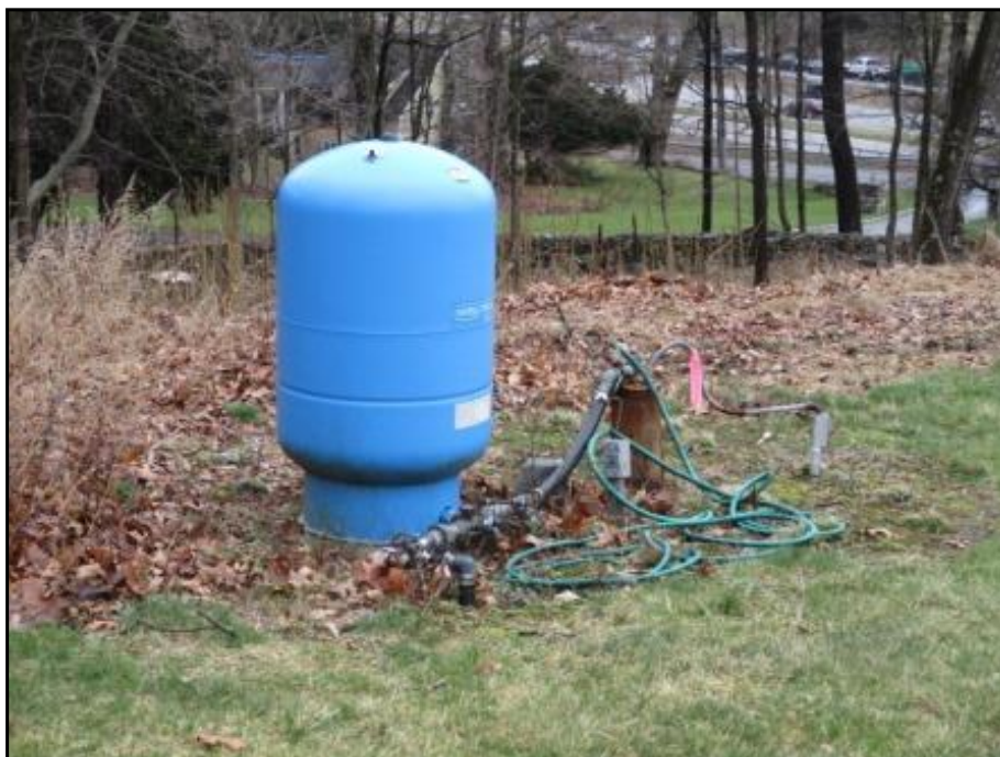
28 : Out-of-service irrigation well on Site
