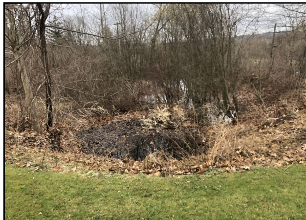
Stormwater retention pond
