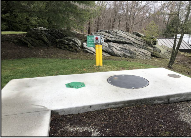
2,000-gallon fuel Oil UST for Building No. 1
