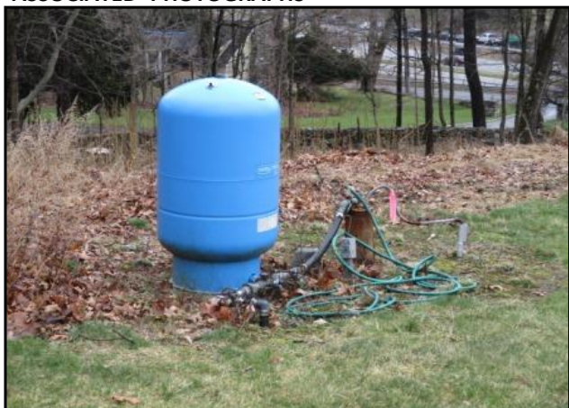
Out-of-service irrigation well on Site
