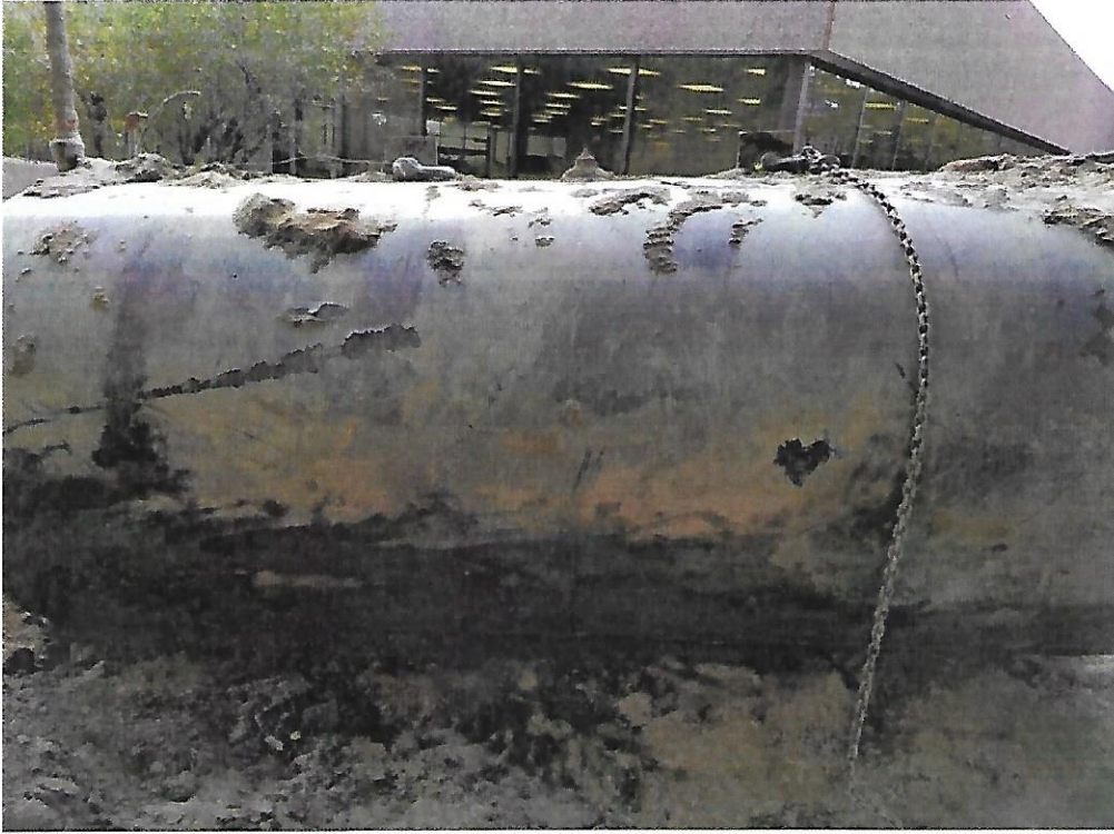
Photograph 3- Another view of tank, no holes or pitting present.
