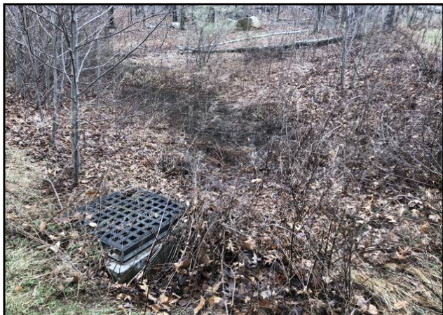
Stormwater retention pond
