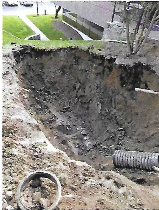
Photograph 4- Tank excavation with tank removed.
