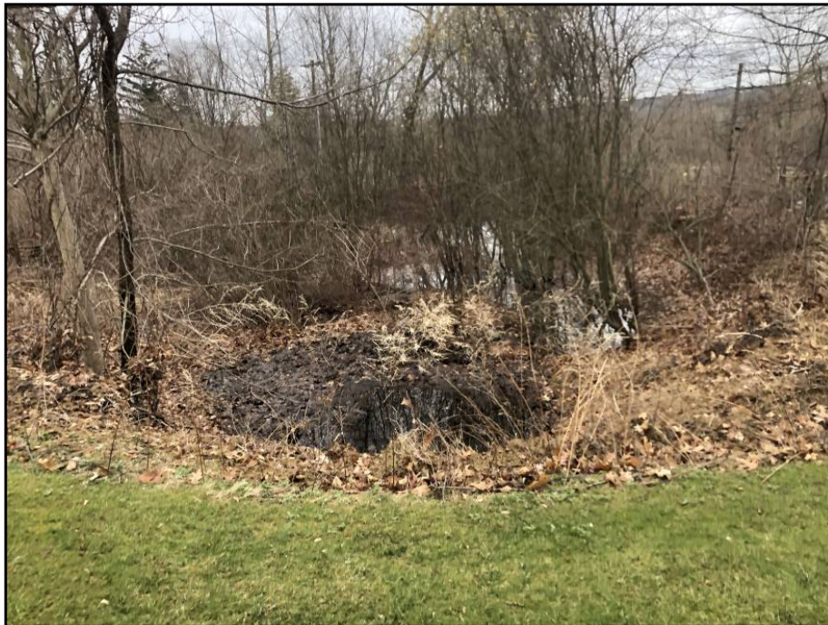
32 : Stormwater retention pond
