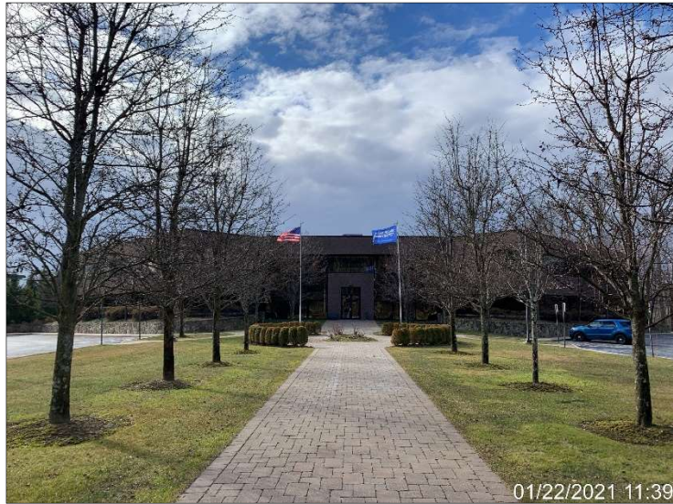
Photograph 13. Building 2, viewed looking southwest.
