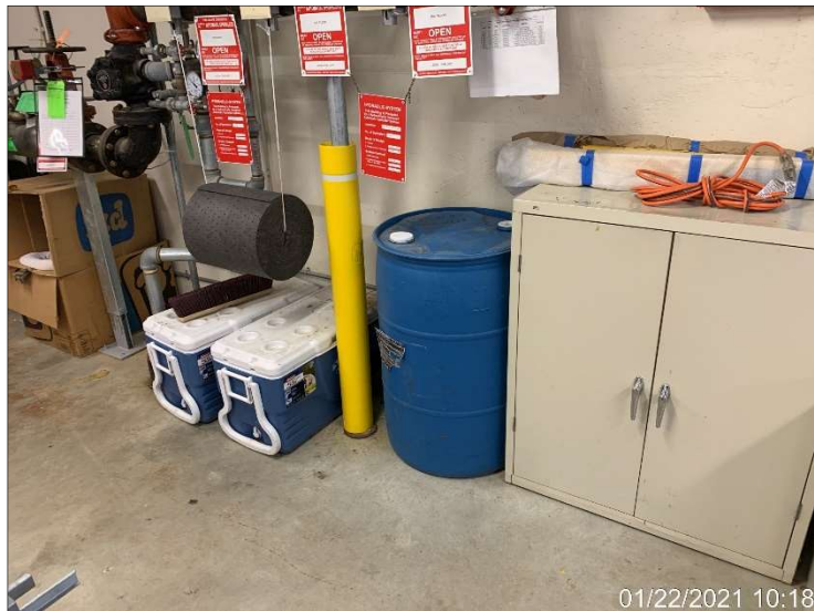
Photograph 15. 55-gallon drum of antifreeze in a maintenance storage area in the cellar of Building 2. The antifreeze is reportedly used in Buildings 1 and 2 to prevent frozen pipes in the heating/cooling systems.
