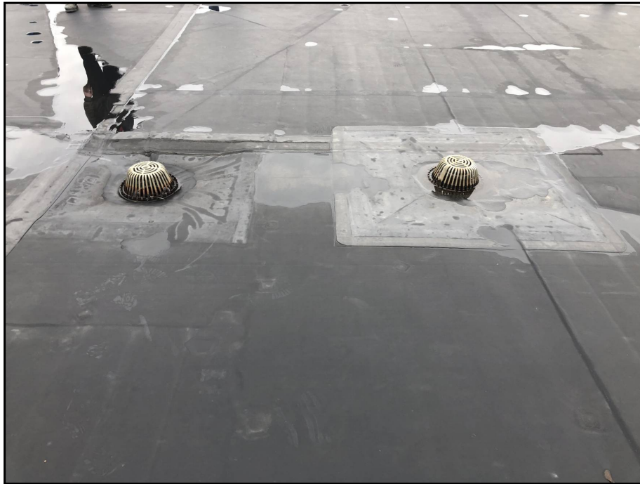
25 : Rubber roof membrane of Building No. 2
