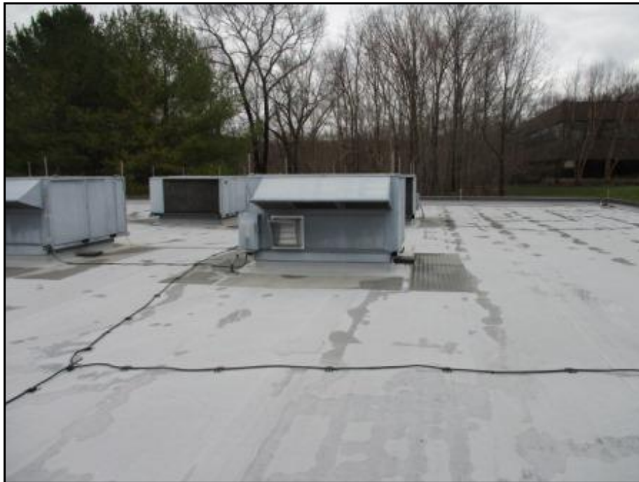
26 : Plastic roofing membrane of Building No. 1
