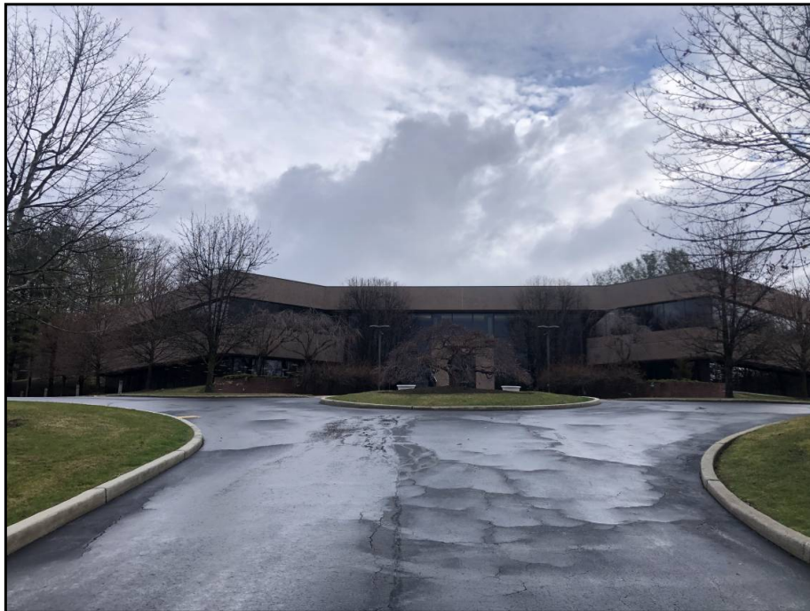
2 : North elevation of Building No. 1
