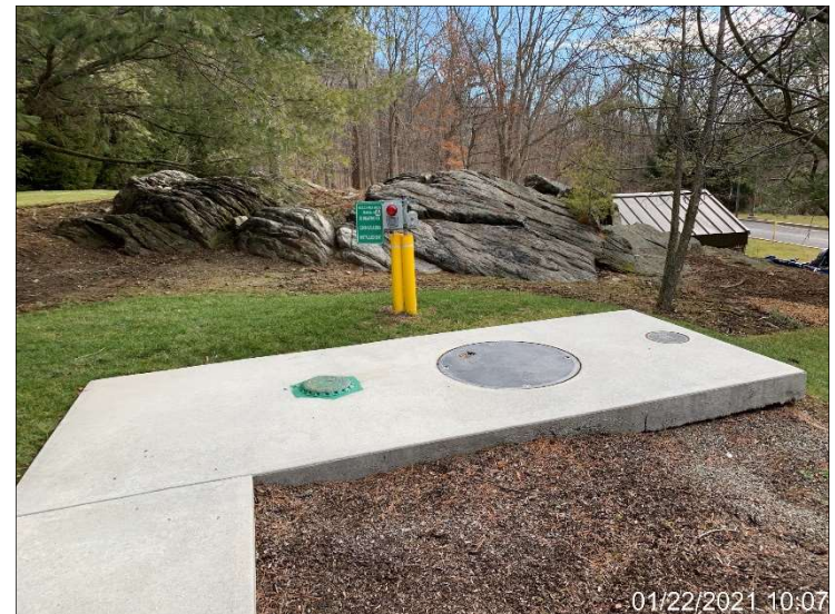
Photograph 8. 2,000-gallon No. 2 fuel oil tank (Tank No. 006) serving Building 1, located outside the northeastern portion of the building.
