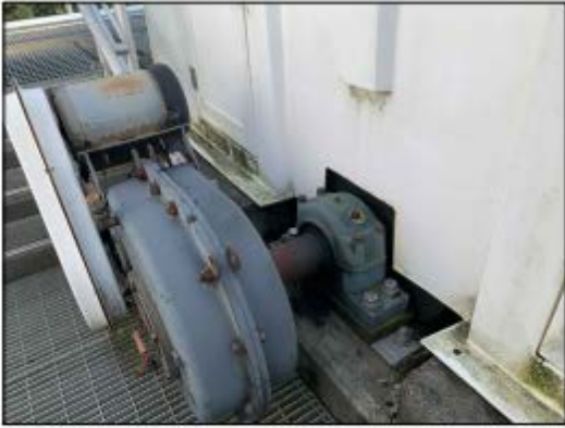
TYPICAL DRIVE BEARING
