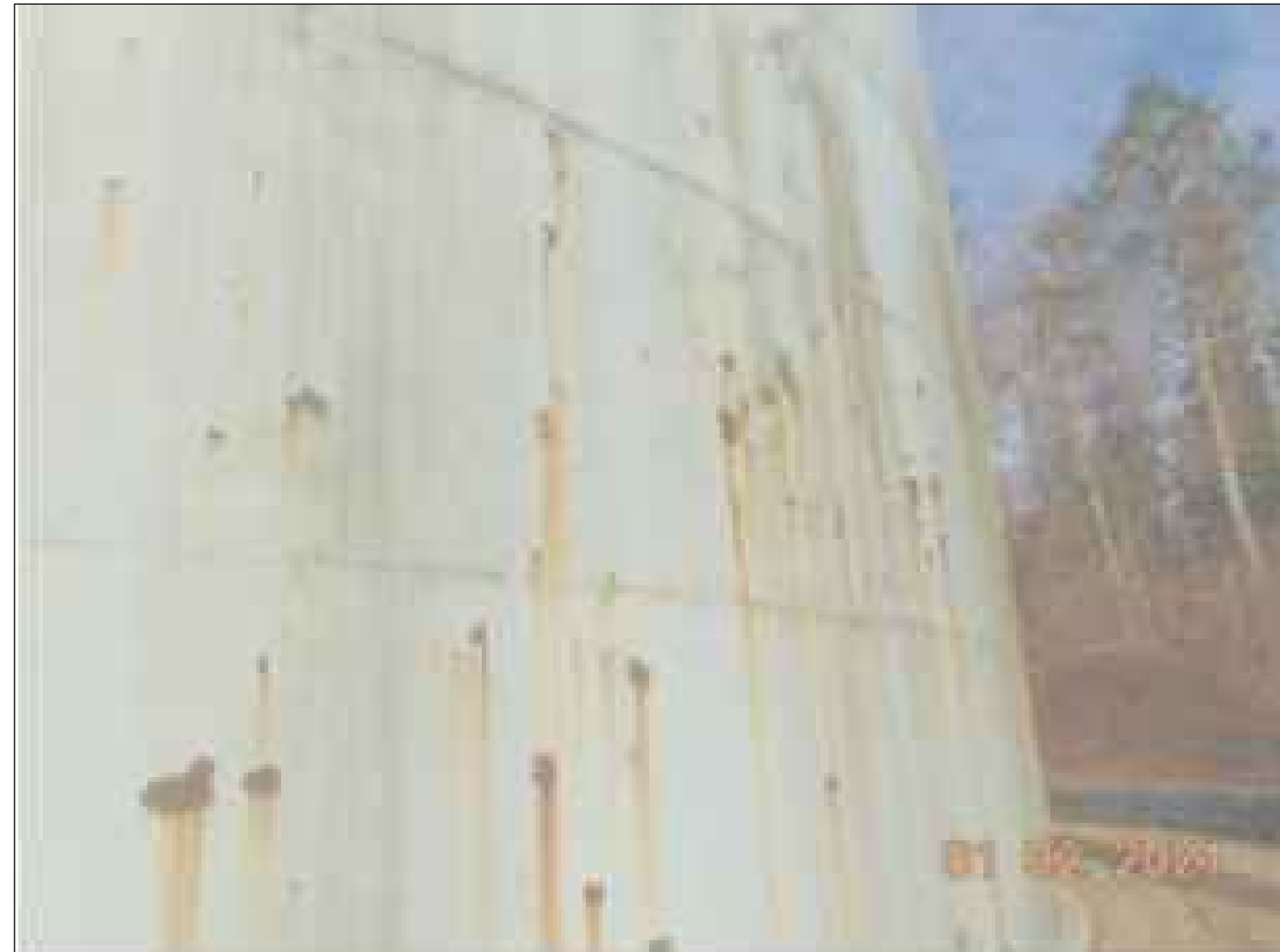
6 CORROSION ON SHELL NOT TO SCALE
