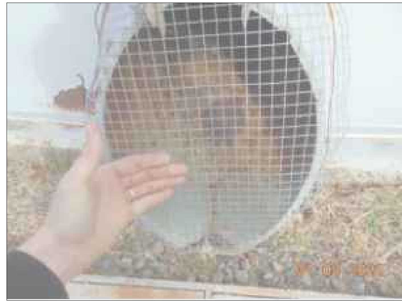
1 OVERFLOW SCREEN NOT TO SCALE
