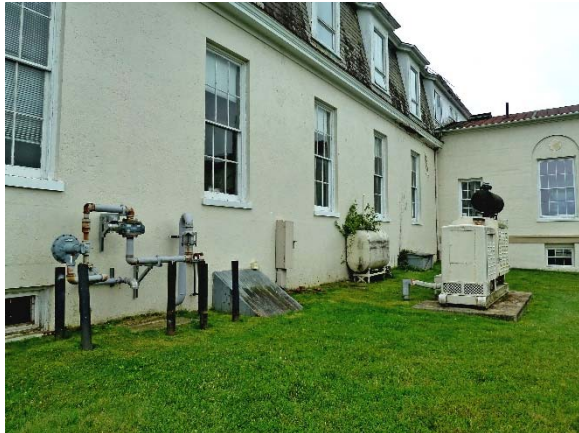
Chapel, north elevation: various utilities, tanks, services present along this façade/lawn
