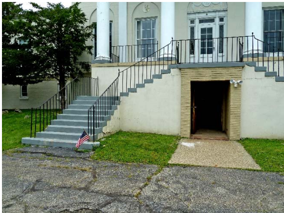
West Addition (1924) allows accessible exterior entry directly to basement level, with exterior stairs to the first floor
