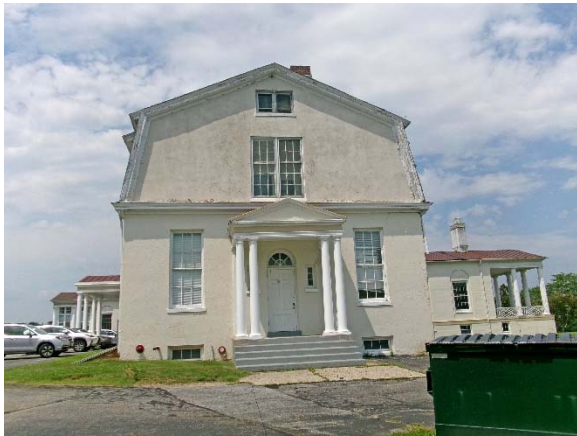
Chapel (1889), east elevation with small porch supported by paired Tuscan columns; portico and pavilions in the distance
