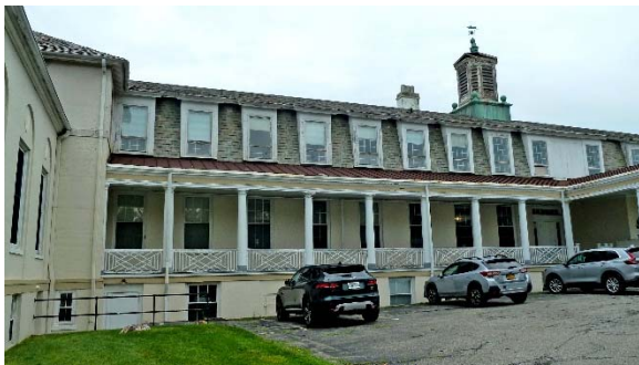
Central Addition (1897): porch in fair condition with likely original standing seam roof, replacement balusters, parking
