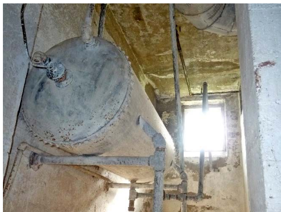
East Pavilion basement: likely remnants of 1924 systems
