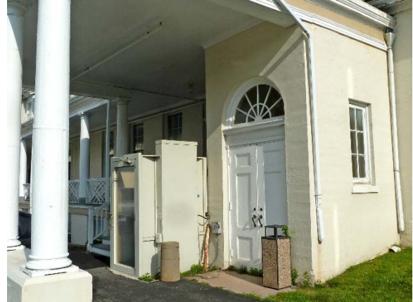
Entry portico (1924 Addition): lift to porch/first floor level adjacent to vestibule leading to Chapel (all beneath roof)
