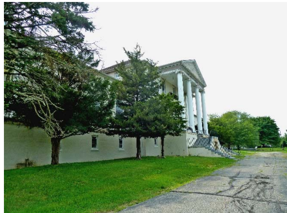
Driveway along formal entry at 1924 Addition, looking southward
