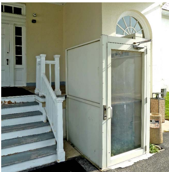
Stairs and lift (possibly inoperable) beneath entry portico, providing access to porch/first floor level
