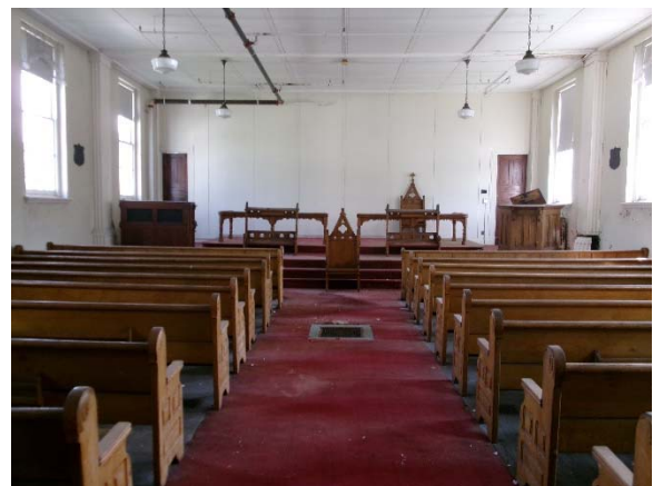
Chapel above basement mechanical room: floor registers in central aisle
