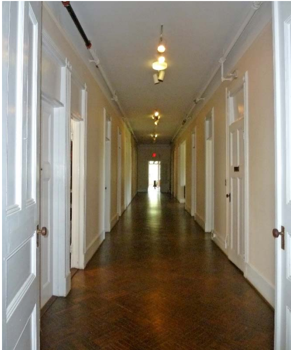
Central hall looking from stair hall outside Chapel westward to main entry vestibule: good condition and currently in use
