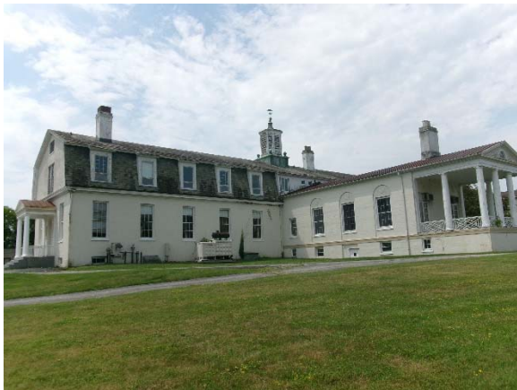
Chapel (1889), north elevation with East Pavilion (1924); driveway encircling the building visible
