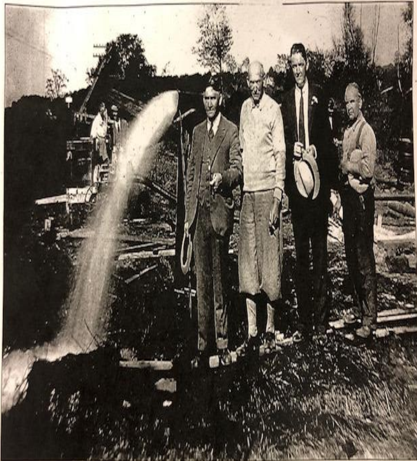
Public water came to Yorktown in 1930. The commissioners of the water board are, from left to right, Samuel S. McBride, Mortimer F. Mckeel, James H. Harding, and Edward L. Dunning.
